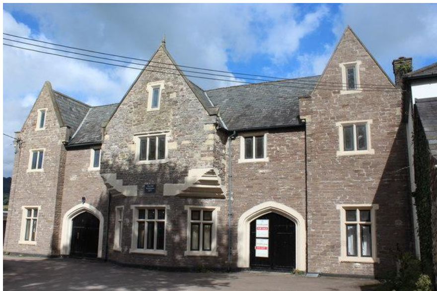
This is what the workhouse building looks like today
